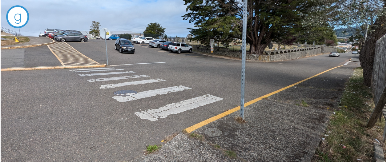
The existing crosswalk over the bus lane and Ingersoll Avenue is missing curb ramps. Half of the crossing (from school grounds to curb median) is currently using loading zone pavement markings. Location: Ingersoll Avenue.
