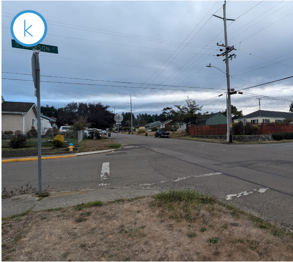
There are missing curb ramps and missing sidewalks along both sides of Pacific Avenue. Students walk in the traffic lanes of Pacific Avenue, versus using the unimproved, often grassy, right-of-way. Location: Pacific Avenue and Madison Street.
