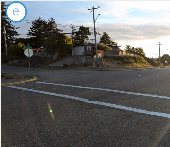
Missing crosswalk on the north leg of the intersection. Faded crosswalk on the west leg of the intersection. Michigan Avenue/South Main Street intersection.
