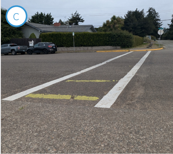
Missing curb ramps on the north leg and the west leg of the intersection. Location: Michigan Avenue/South Main Street intersection.
