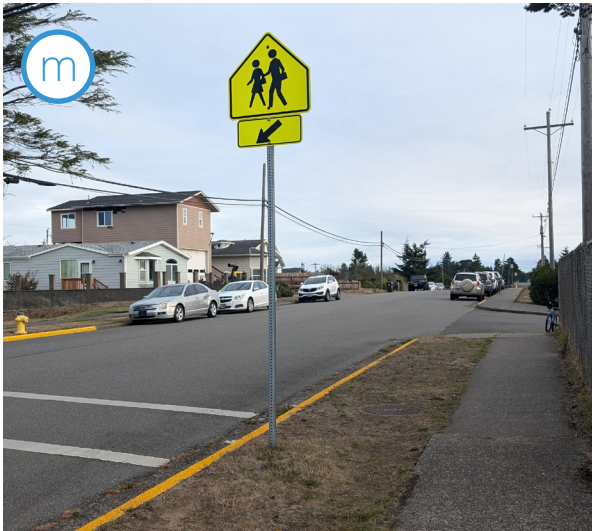
There are missing curb ramps and missing sidewalks along both sides of Pacific Avenue. Students walk in the traffic lanes of Pacific Avenue, versus using the unimproved, often grassy, right-of-way. Location: Pacific Avenue and Madison Street.
