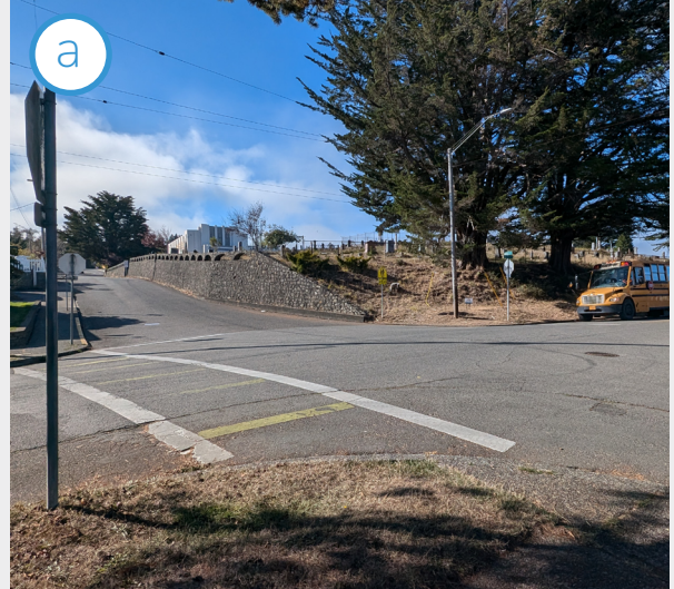
There are missing curb ramps, as well as missing or faded crosswalks at numerous key intersections close to the high school. Location: Ingersoll Avenue and S. 7th Street intersection.
