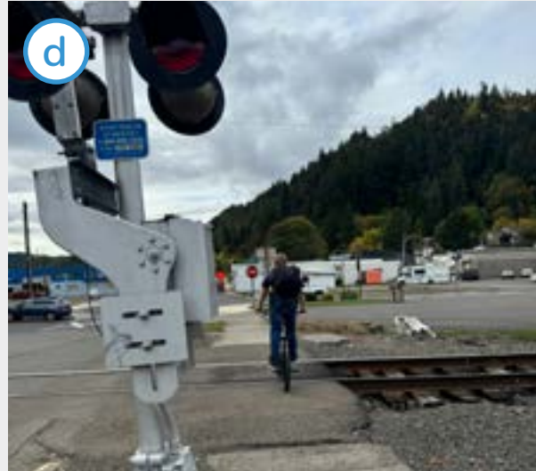
Unmarked pedestrian railroad crossing on East B Avenue. Additionally, the vehicle railroad crossing pavement markings are faded. Location: East B Avenue.
