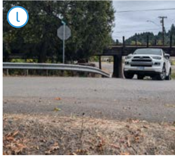
Westbound vehicles on Moreland Avenue pull up beyond the stop line to see around the blind corner that is created by the bridge on 1st Street. Pedestrians cross to this corner as well as from the sidewalk on the opposite (west) side of the bridge to walk through the railroad undercrossing. Location: South 1st Street and Moreland Avenue intersection.
