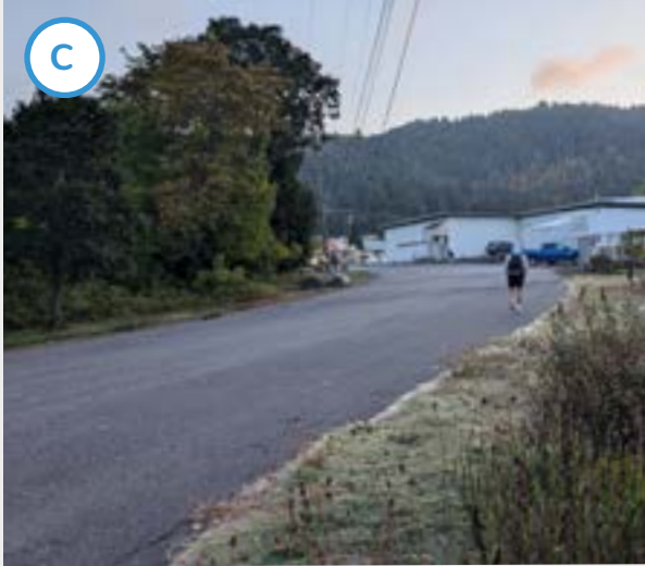
There are missing sidewalks along Moreland Avenue, from the railroad undercrossing to Hendrick Creek Avenue. This is a popular route for students walking to the high school.
