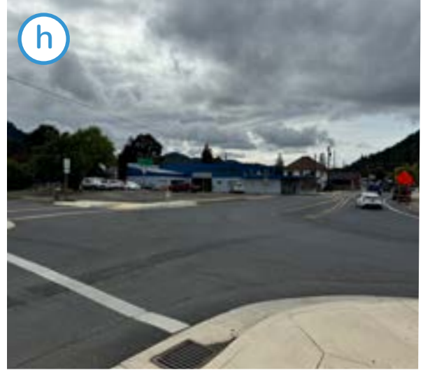
The Highway 38 curve north is poorly marked for eastbound traffic, resulting in confusion for vehicles continuing east instead of turning north. Location: West B Avenue/North 1st Street intersection.
