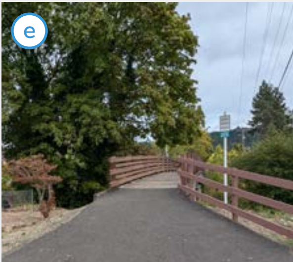
Students use the existing footbridge over Elk Creek to reach the other side of Drain. There are missing sidewalk connections along Payton Avenue to this bridge.
