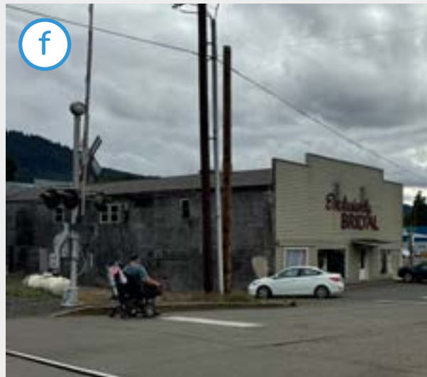
Missing sidewalk on the south side of East B Avenue from 117 East B Avenue to the intersection of East B Avenue and North 1st Street, near the bridal shop. Location: East B Avenue.
