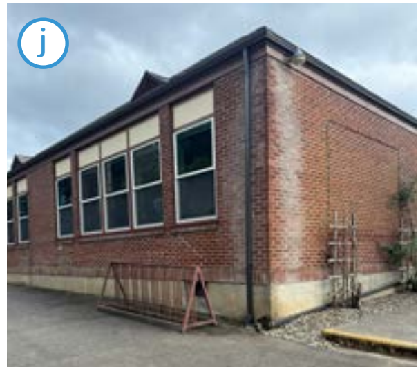
There is one existing bike rack located on the north side of the elementary near the front entrance. It is uncovered, and the design is not user friendly.
