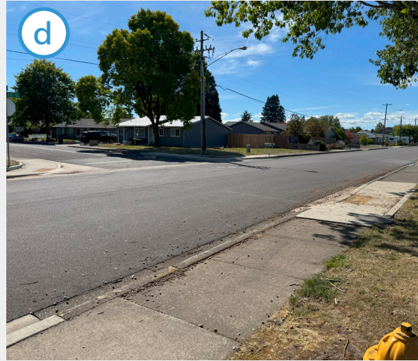
Existing ADA ramp crossing of LaSalle Street south of Harrisburg Elementary lacks signage and striping.
