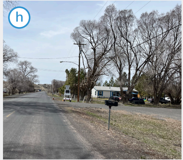
The Tribe's previous transportation plan designated shoulders along the roadway as bike/ped facilities; However, these are not clearly marked and have no separation from vehicles.
