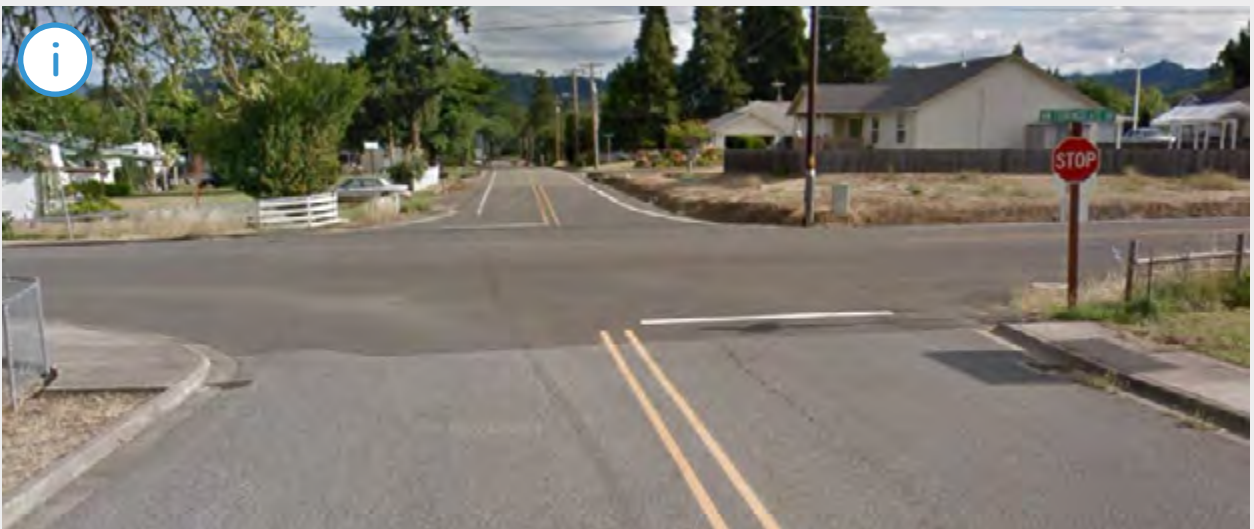
The intersection of NW Brockway Rd and Lookingglass Rd does not have a marked crosswalk or curb ramps on three corners. This intersection separates a major neighborhood from the school. There are sidewalks on the north side of Lookingglass that end on the east side of the intersection and there are sidewalks on the west side of Brockway Rd. A crossing at this intersection would connect these two sidewalk facilities.
