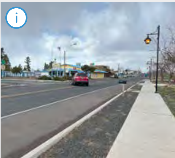
New sidewalk, lighting, and curb ramps on the west side of Culver Highway and E Street.
