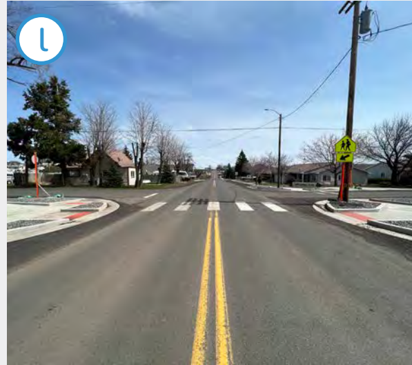
The new curb ramps along Walnut St no longer align with the crosswalk markings at Lincoln St.
