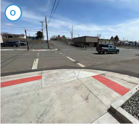
The intersection of Main St and Spring St has new curb ramps but lacks continental-style crosswalk markings.
