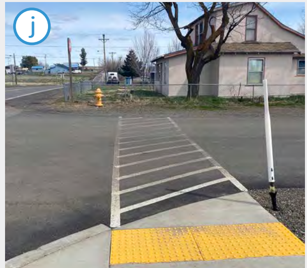
The current crossing of the south leg of the intersection of E Bayard St and Washington St is missing a curb ramp on the east side.
