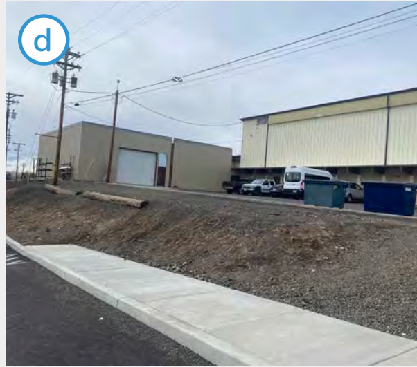
Referred to by some as the "Condon Cliff," this slope exists on the south side of Condon High School. The base of the sidewalk at the crossing lacks a curb ramp, because its not an accessible route due to the steepness of the sidewalk to the east.
