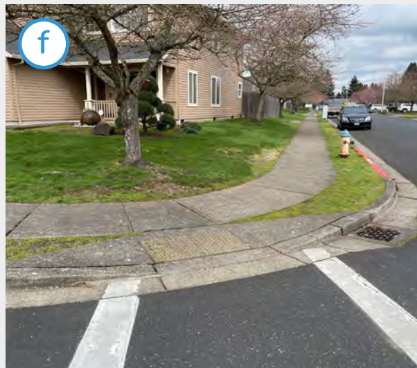
The pedestrian path connecting Grant Watts and Otto Petersen Elementary Schools continues north on a multiuse path. This path crosses SE June Ln, where there is a parallel bar marked crosswalk. On approach to the northern sidewalk, there is an irregular curb ramp.
