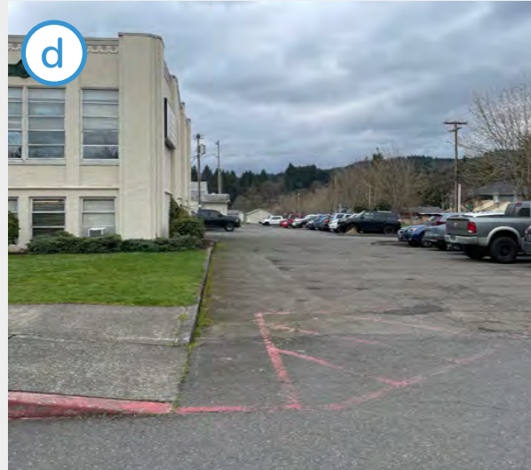
The Scappoose Middle School parking lot is located on the north side of the school. The pavement markings are faded in some locations.
