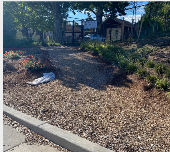
The bark path at the entrance to trail at north side of campus is made less accessible by the presence of the concrete curb.
