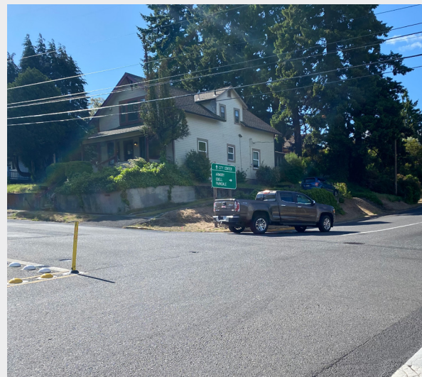
There are missing sidewalks and curb ramps at the southeast corner of May St and 13th St. Existing ramps at this intersection are considered "poor functional condition", according to ODOT's ADA inventory.
