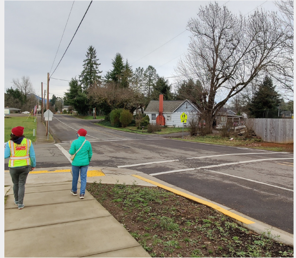
The intersection of 22nd Ave and Mountain View Rd currently features three crosswalks with transverse markings. The only ADA-compliant curb ramp is on the southwest corner.
