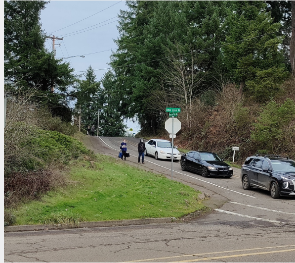
Mountain View Road is steep and winding, which reduces visibility along the corridor. There are currently no sidewalks or bicycle facilities. The intersection has minimal lighting, poor sight lines, and high volumes of vehicle traffic.
