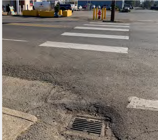
At the intersection of Church St and Hwy 219 / Main St, some curb ramps have been updated to comply with ADA standards, but others are not improved. In some cases, storm drains are located near where curb ramp improvements are needed.
