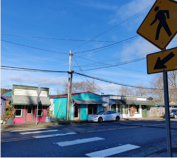
The existing marked crosswalk in downtown Cloverdale, located midblock between Bridge St and Campground St, is faded and not highly visible.
