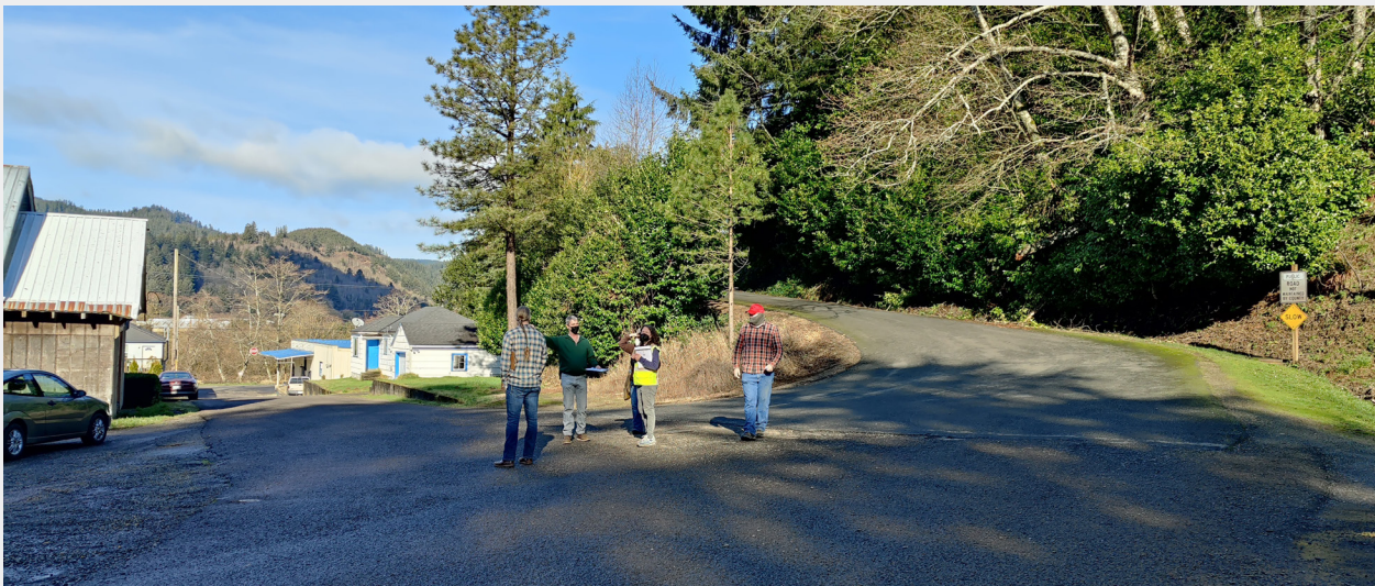
The intersection of Brook St and Campground St is large, expansive, and undefined. It has no traffic control devices or road striping. Students wait for the school bus at the gravel area along the northwest corner of the intersection. Lack of pedestrian facilities, poor lighting, and drivers going too fast for conditions create safety concerns for students walking through or waiting in the area.
