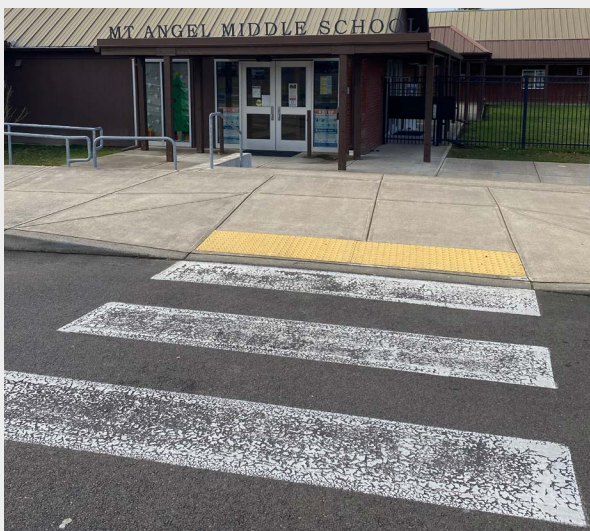
Crosswalk is faded with poor visibility leading from the parking lot to the main entrance of the middle school.
