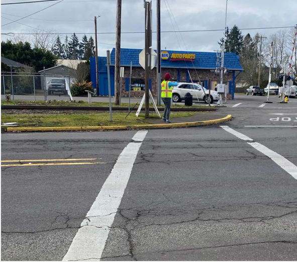
The crosswalk at E Church St and Hwy 214 is faded and lacks ADA-compliant curb ramps. Vehicles are often traveling into town at high speeds on the Hwy 214.
