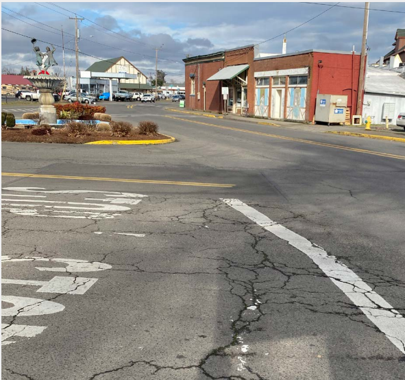
The intersection of E Church St, Hwy 214, and Main St is uncomfortable for pedestrians and confusing for drivers. The crosswalks are faded and not highly visible.
