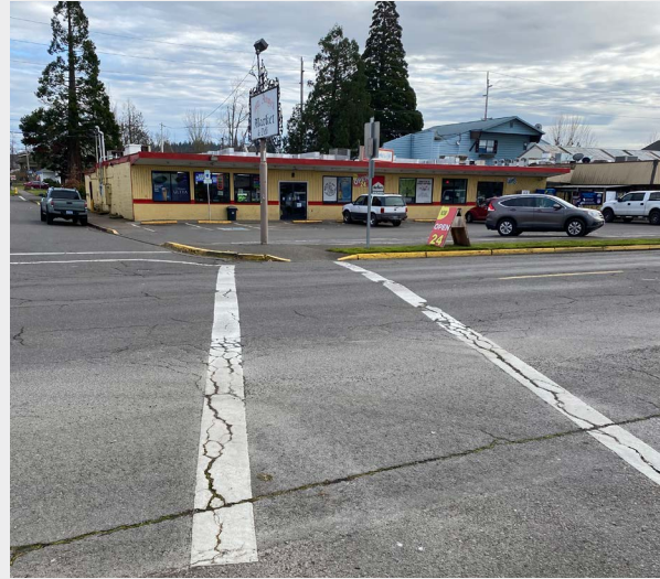
The intersection of Taylor/John St/Hwy 214 is uncomfortable for pedestrians. Vehicles parked at the northeast corner of the intersection on Main St block sight lines. There is a need for enhanced high-visibility crosswalks with improved illumination at this intersection.
