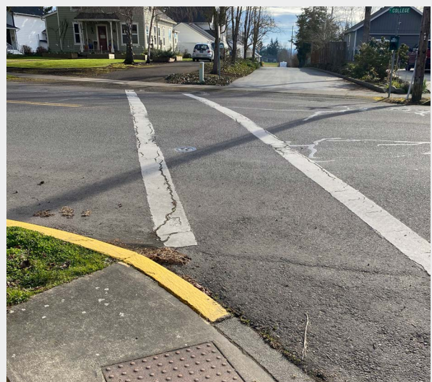
Crosswalks at College St and Elm St are faded and lack high-visibility markings. Student frequently walk in this area and cross both College St and Elm St (from the dirt parking lot across from the school) to reach the St. Mary's School campus.
