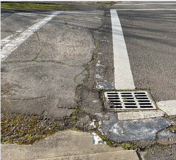
There are damaged curb ramps at the intersection of Elm St and Taylor St.
