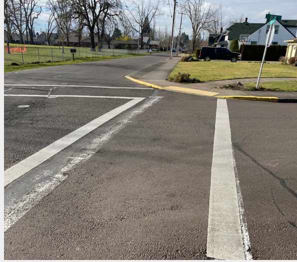
The intersection of Elm St and Taylor St is frequently used by students. The crosswalks are not high-visibility and lack ADA-compliant curb ramps.
