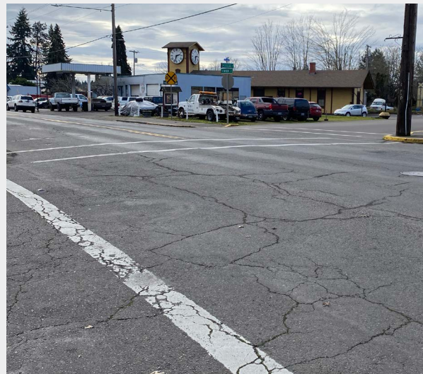
Crosswalks at the intersection of College St and Main St are faded and poorly visible.
