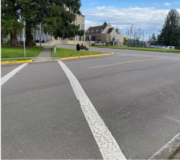
The crosswalks at Oak St and College St are uncomfortable for pedestrians. Two crosswalks are very close together across Oak St, and there are poor sightlines.
