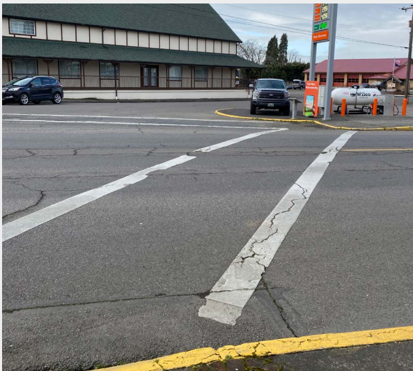
The crosswalk at E College St/Hwy 214/Monroe St is faded and lacking ADA-compliant curb ramps.
