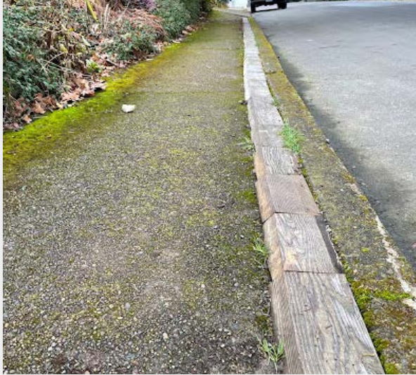
Sidewalk conditions are poor along Jackson St, near the Heffley St/Jackson St intersection. Sidewalks are also not ADA-accessible.
