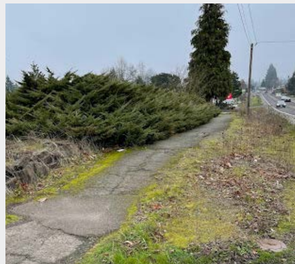
The sidewalks along Main St at Heffley St are not well-maintained, creating a barrier for students walking and rolling along this route to school. The slope is also very steep, causing visibility issues. Additionally, public transit cannot provide bus stops along the section of Main St from Heffley St to the "S" curves due to the separation of sidewalk and roadway, as well as the non-ADA-compliant nature of the sidewalks.
