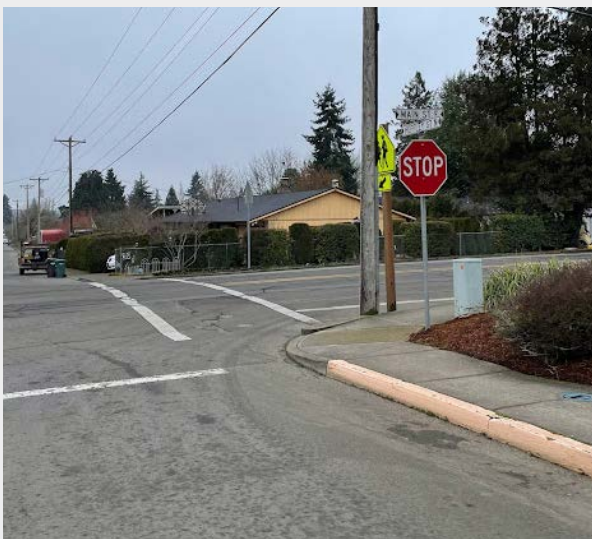
The Heffley St and Main St intersection is a busy pedestrian and vehicle area. There is only one crosswalk here (not high visibility), and the stop lines are faded on the northern and southern legs of the intersection.
