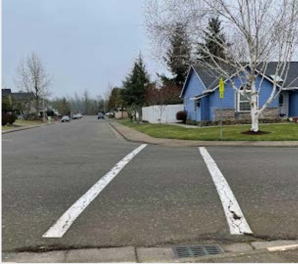
The crosswalk at the intersection of Kayla Way and Margaret St is faded and lacks ADA-compliant curb ramps. This is a crucial crosswalk for students accessing the pedestrian path to campus.
