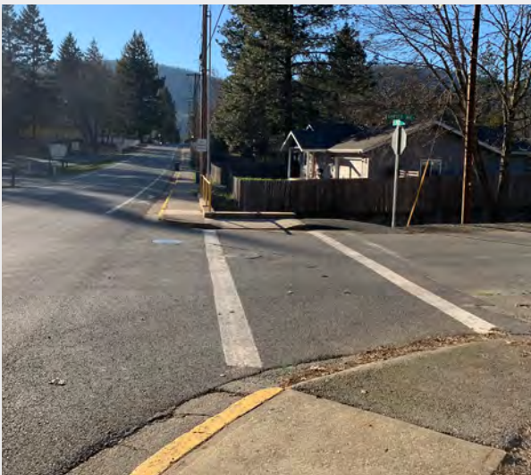
Curb ramps along this route are not ADA-compliant.
