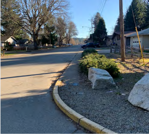
Curb ramps are missing along River St, making it difficult for people with mobility limitations to navigate the pedestrian facilities.
