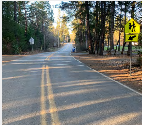
Old Stage Rd has no pedestrian facilities. There is a crosswalk with school crossing signage, but it is not connected to any established east-west pedestrian facilities. There is a pathway that students use as a most direct route to school, but it is overgrown and on private property.
