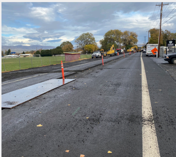
Hostetler St is currently under construction for utility repair. Students can connect to a paved path that leads to the school from the southeast corner of the property.
