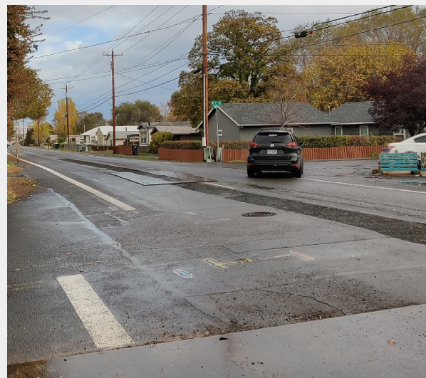
7th St is a major north/south route that students use to get to school.
