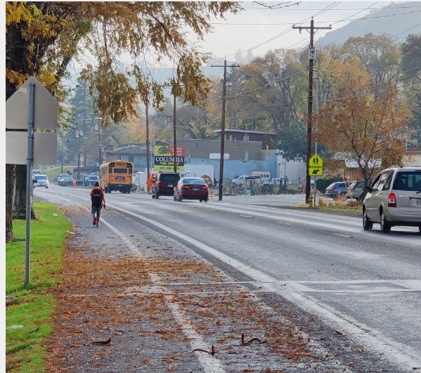
Lack of sidewalks on 10th St between Chenoweth Loop Rd and Hostetler St forces students to walk on the shoulder.
