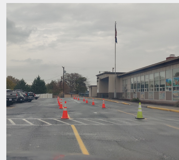
The Chenoweth Elementary parking lot was reconfigured to include multiple queuing lines in order to reduce backed up traffic on Chenoweth Loop Rd.
