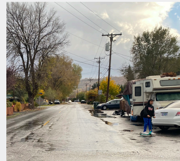
Looking southward on 7th St from Hostetler St, one can see the lack of sidewalks and undefined edges on both sides of the roadway, forcing students to share the roadway.
