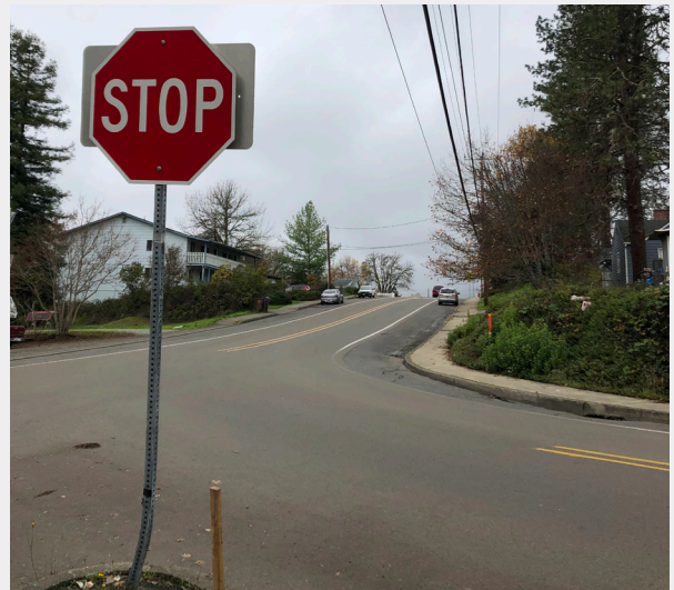
The existing configuration of the intersection allows vehicles to turn from Myrtle Rd onto Division (and vice versa) without stopping. Higher speeds, combined with short sight distances, lack of sidewalks, curb ramps, crosswalks and signage creates a significant barrier for people walking and rolling.
