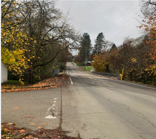
Further east on Division St, the sidewalks end and the narrow roadway width with steep drainage ditches force bicyclists and pedestrians to share the roadway. The bridge over Myrtle Creek has a separated sidewalk on the south side.
