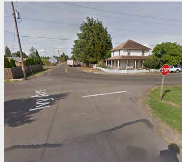
At Ivy Ave and 3rd St, trucks turning SW from Ivy Ave onto 3rd create a hazard when they have to make wide turns into the NE-bound lane. This creates a barrier for vehicles traveling NE on 3rd, who are unable to see the trucks easily.
