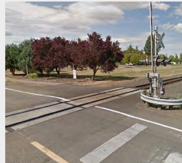
The at-grade railroad crossing west of 4th St lacks clear signage and markings indicating where pedestrians should wait when a train is approaching. The existing sidewalks do not connect all the way over the crossing.
