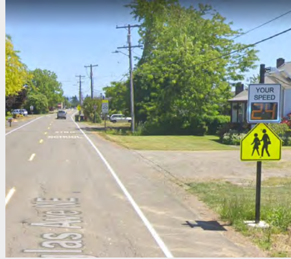
While there is a radar feedback sign and school zone sign warning drivers to slow down, these signs are routinely ignored, creating a potential hazard for people crossing near the elementary school.
