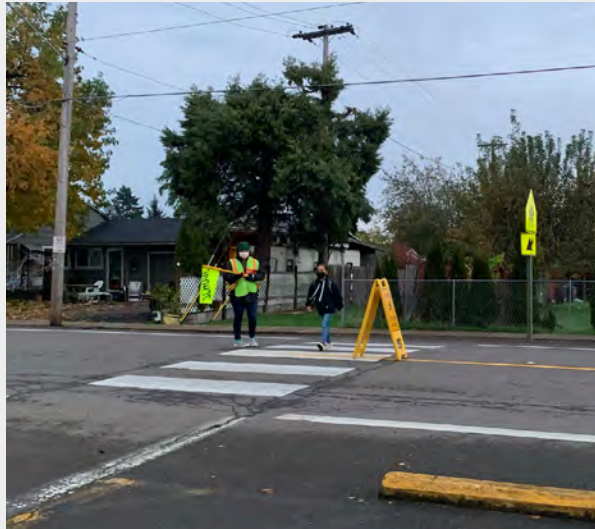
The school crossing is located at mid-block on Douglas Ave between 2nd St and 1st St. This is not an ideal location for visibility and creates an additional required stop for vehicles traveling along Douglas Ave.
