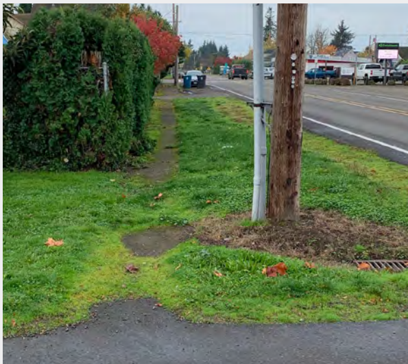
Sidewalks along 3rd St have many gaps. There are also obstacles present, such as utility poles, overgrown grass and moss, broken and uneven concrete, and puddles, which limit how accessible the sidewalk is for people of all ages and abilities.
