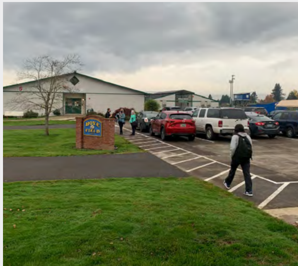
The middle school parking lot has designated pedestrian travel paths marked on the pavement.
