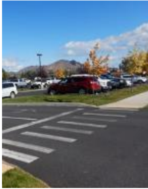
Crosswalk paint is faded and some lack curbs and tactile paving.
