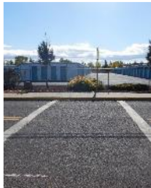
Crosswalk paint is faded and some lack curbs and tactile paving.
