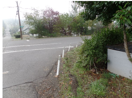
Looking south, NE Cypress St and NE 5 th Ave intersection. Bollards mark the edge of the roadway to prevent vehicles from cutting the corner on this frequent walking route.
