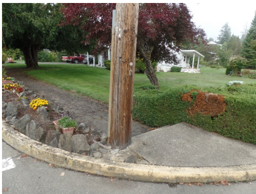
Looking west, Oak St and NE 5 th St intersection. All curbs lack ADA-compliant curb ramps and some corners include utility complications.
