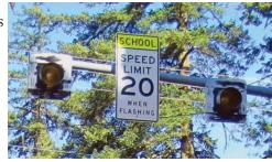
School beacons should be placed on or immediately adjacent to the School Speed Limit sign assemblies with the "WHEN FLASHING" plaque. See *Section 4L.04 of the MUTCD*.
